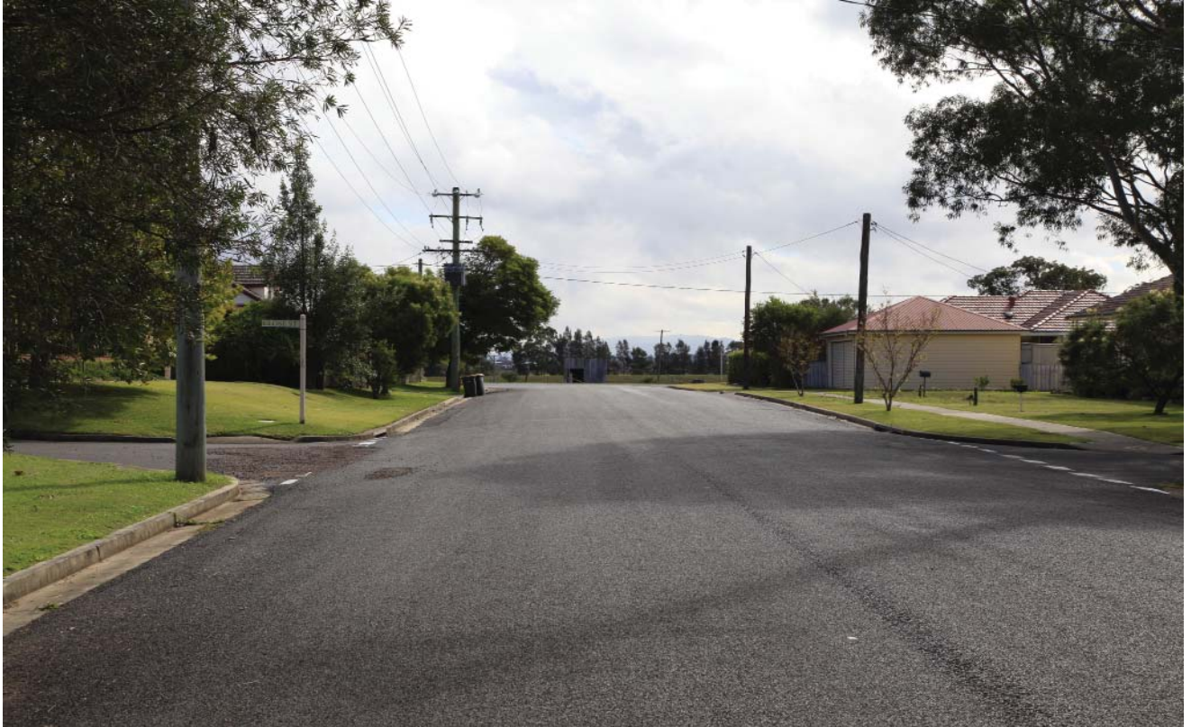
Location 5: Axial view north along Edward Street from south of its intersection with Close Street.
